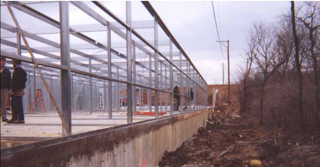
A finished stemwall.
