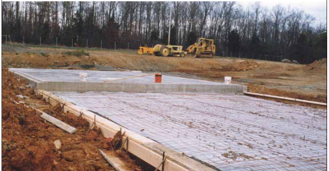
Each section of foundation is poured to the next step.
